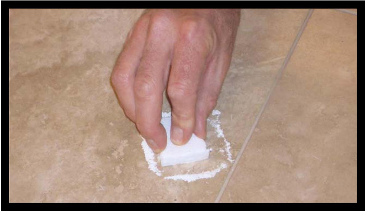
**Step 7:** Using small circular motions pack the grout into the wet hole. The water that is already in the hole and surround stone will set the grout.
