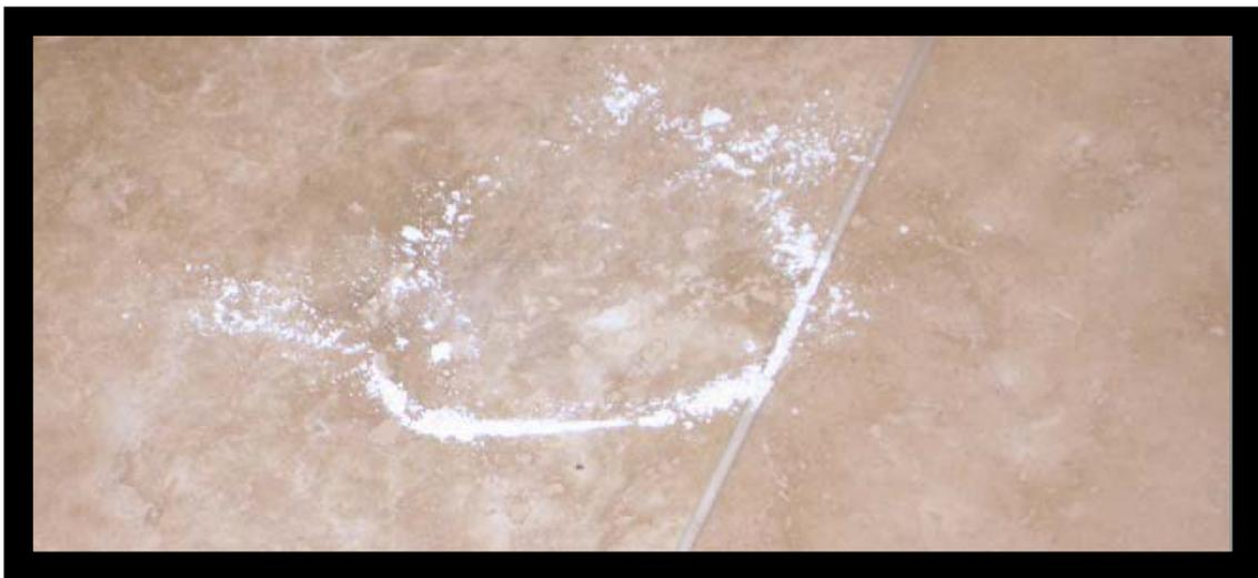
You will easily realize the same result as above. The void in this example is just off the knife point. The grout will need 8 hours to harden prior to use.
