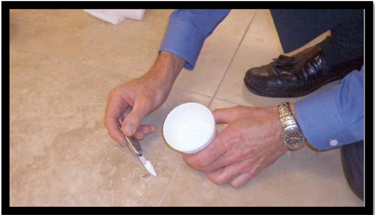
**Step 5:** Using a flat tool such as a screwdriver or a knife put a mound of grout over the void, sufficient to completely fill the void.
