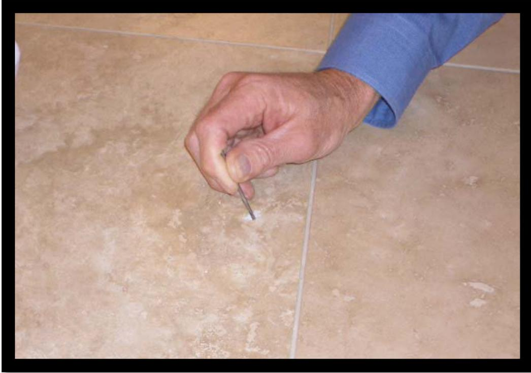
**Step 1:** Clean all debris from void using a small tool to loosen and remove all particles.
